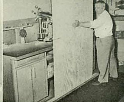
HORIZONTAL SAWING. Tilt motor vertical, set saw parallel to table top and cut across 4 foot wide panels this way. Saw can be lowered or raised for desired width.
